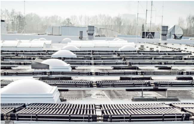
The solar ice system's rooftop solar absorbers
